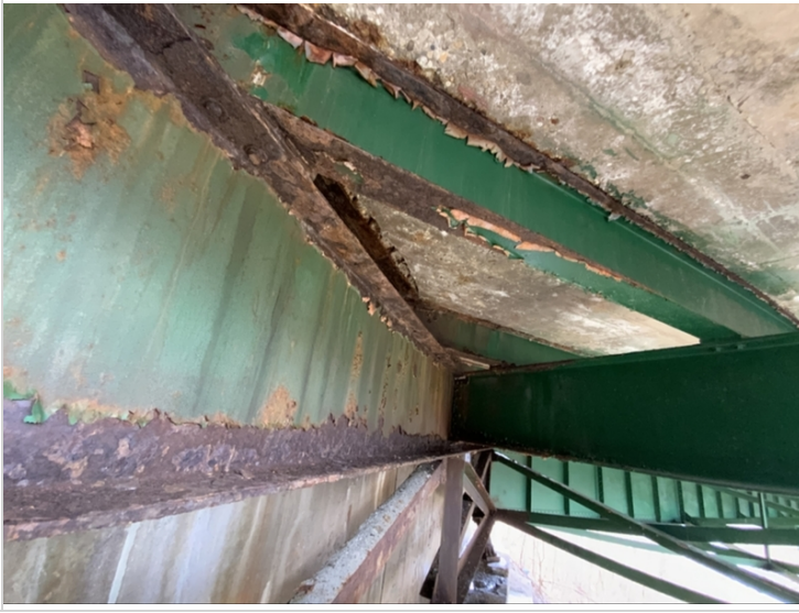
Abutment 1 floor beam and stringer ends
