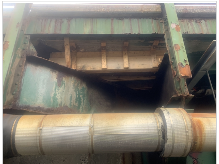
Nail/Screw laminated timber stringers (repair) over abutment 2
