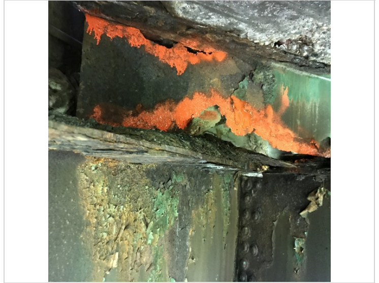
Upstream interior stringer over abutment 2
