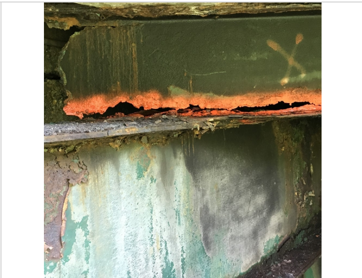
Upstream stringer over abutment 2
