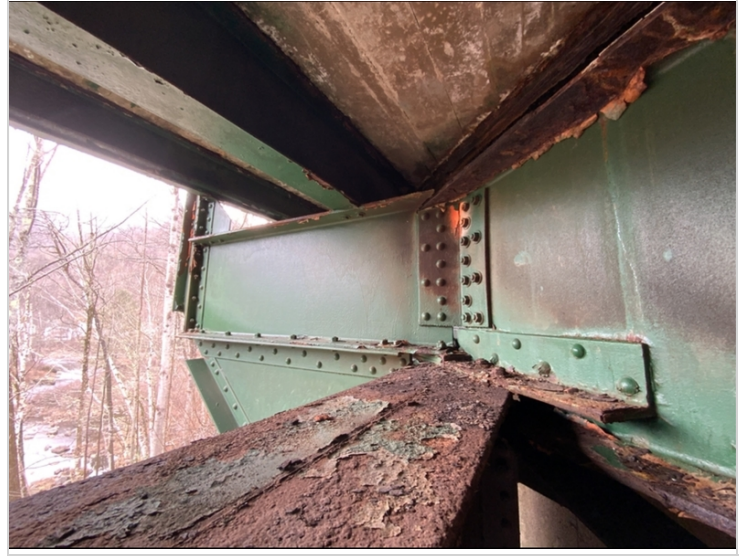
Abutment 1 downstream floor beam extension
