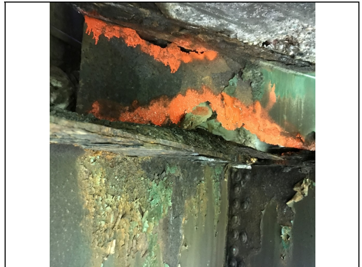
Upstream interior stringer over abutment 2
