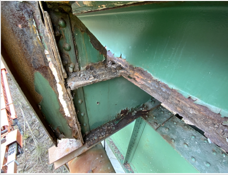
Upstream stringer at floor beam 16
