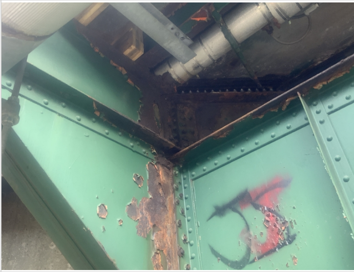
Abutment 2 upstream floor beam extension
