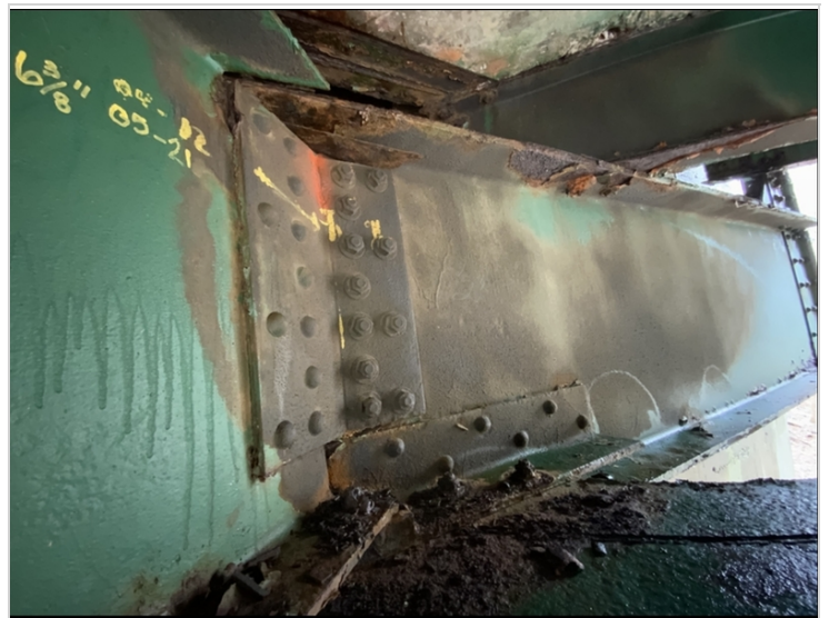
Abutment 2 downstream floor beam extension
