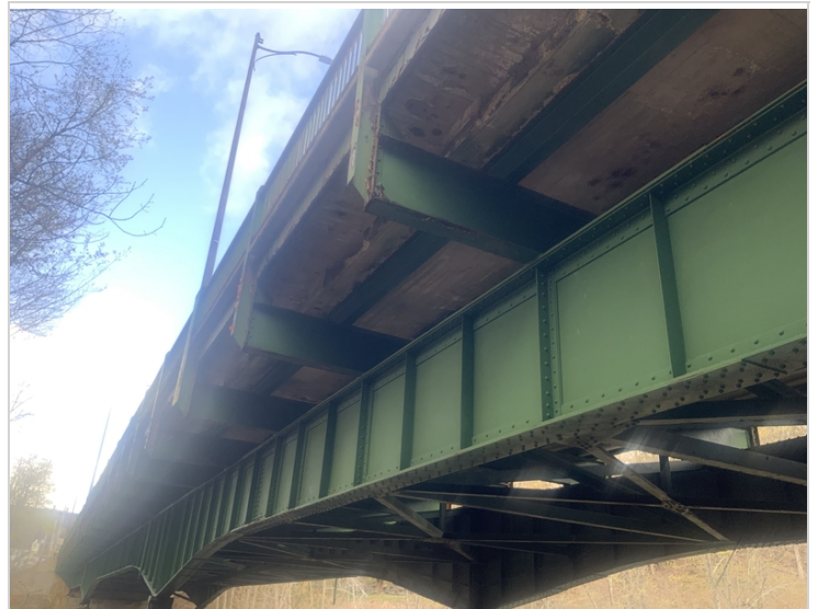
Downstream fascia/Sidewalk soffit
