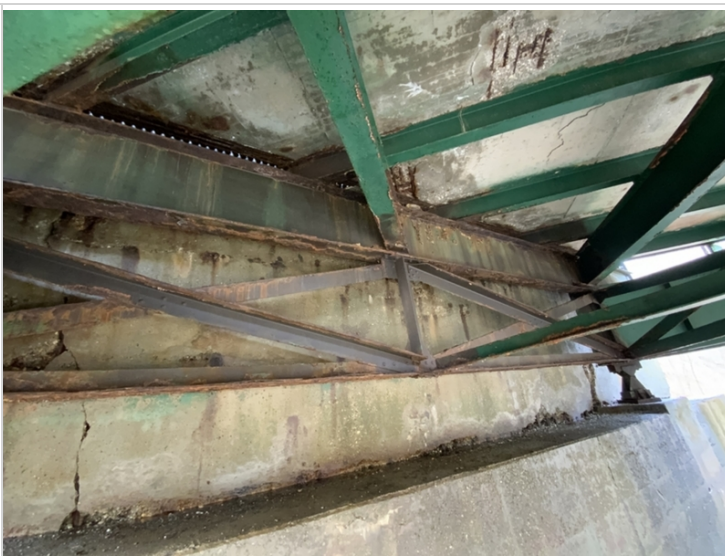
Abutment 2 floor beam and stringer ends
