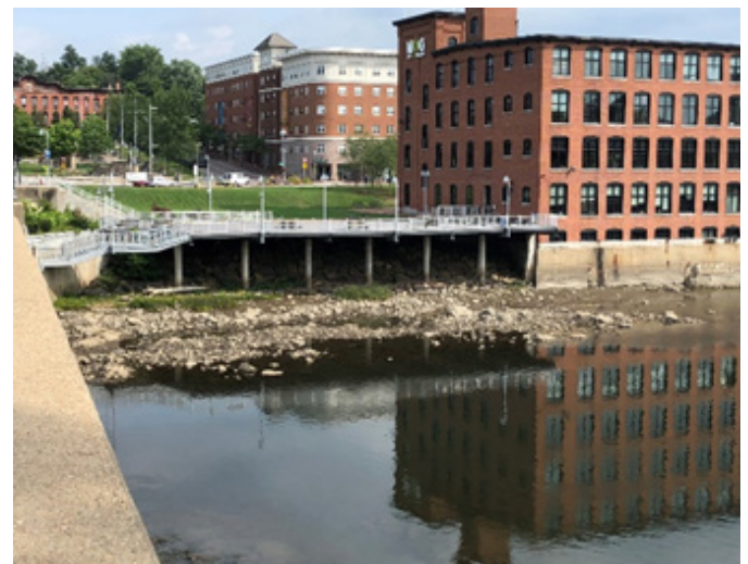
Fig. 11 – Looking North at the Riverwalk Deck and Mill Building
