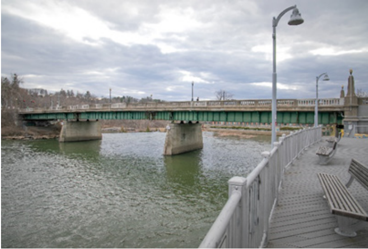
Fig. 6 – Looking West at the Bridge from the Riverwalk
