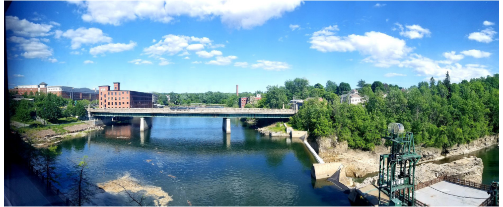
Fig. 1 - Existing Winooski River Bridge Looking East
