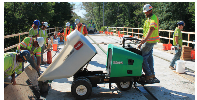
Fig. 24 - Utilizing UHPC Will Reduce The Full Closure Time for Motor Vehicles
