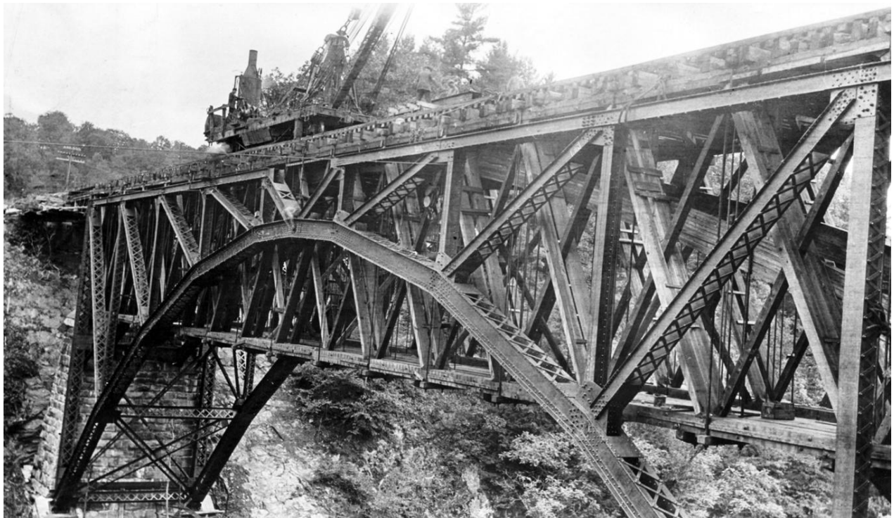
Figure 3. Construction of Bridge No. 61 in 1911.
