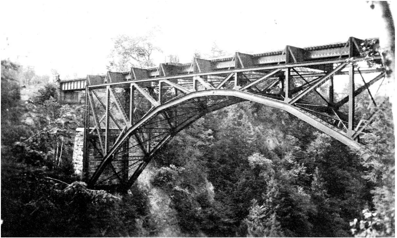
Figure 4. Completed Bridge No. 61 in 1911. Note rail deck.
