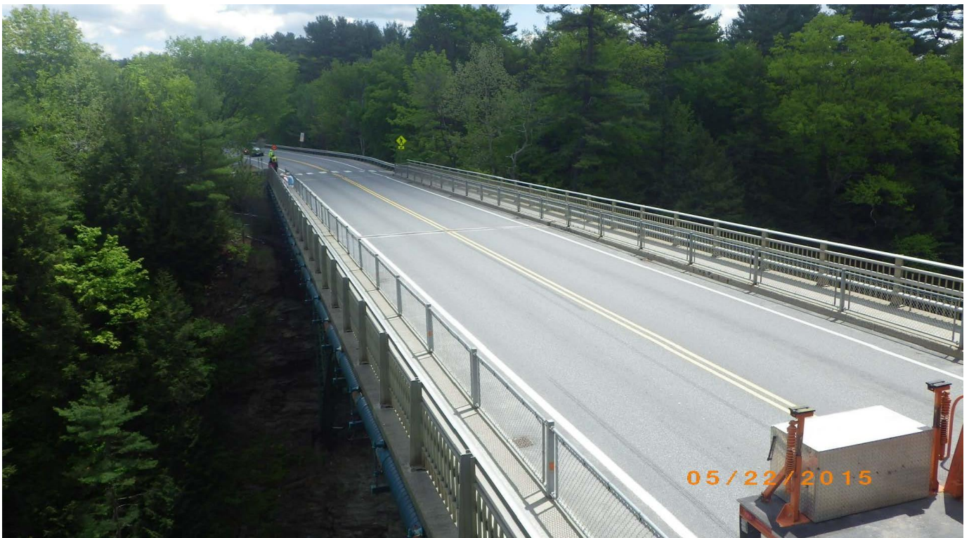
Figure 7. Bridge No. 61 deck, looking west on US Route 4.
