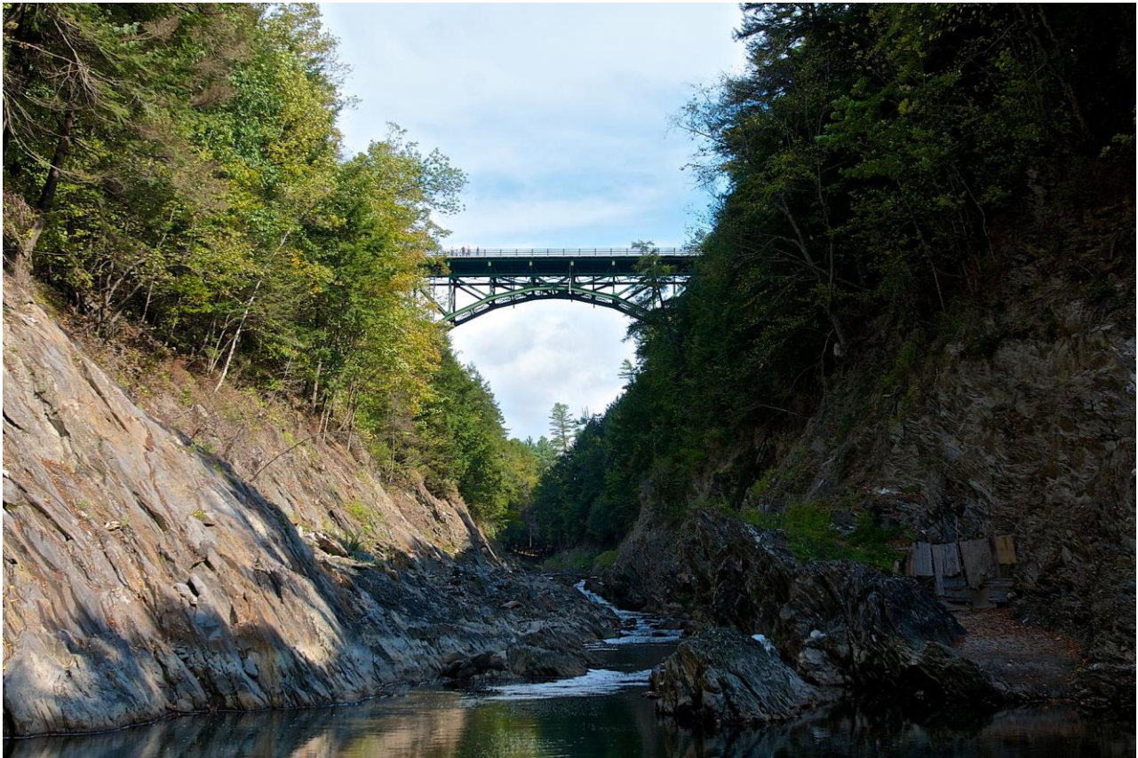
Figure 2. Bridge No. 61, Quebec Gorge Bridge, looking south from the Ottawa-Quebec River.
