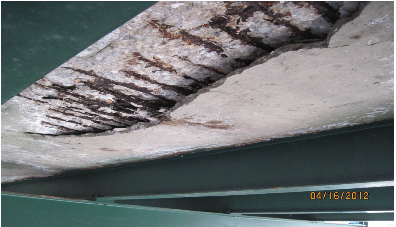
Delaminating Deck
