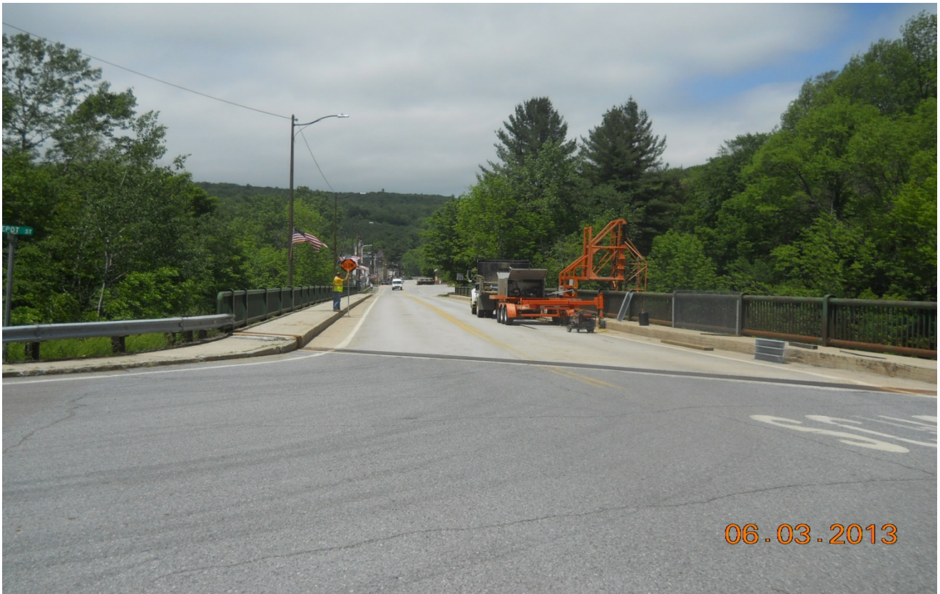
Bridge 25 Looking West
