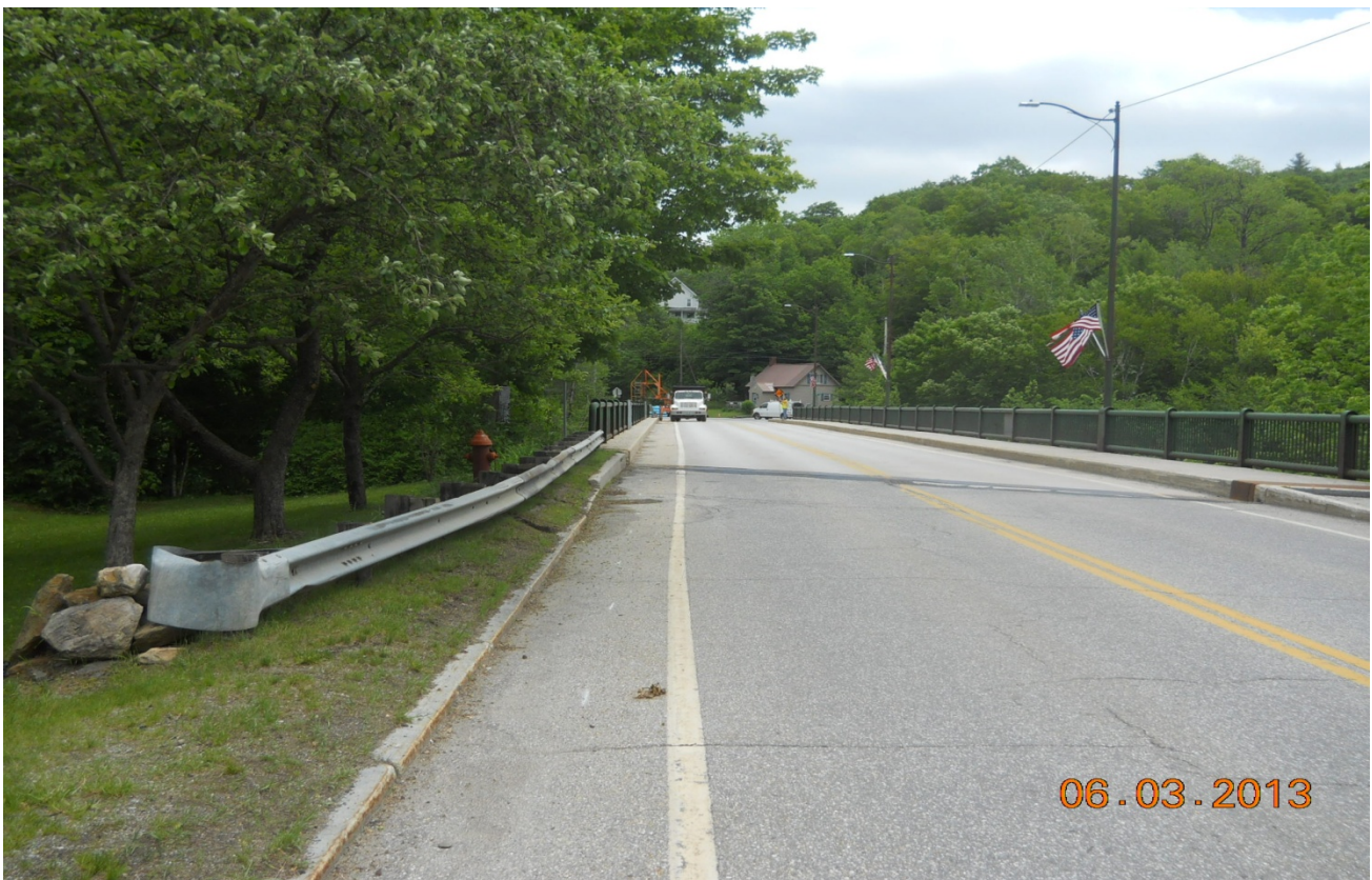
Bridge 25 Looking East
