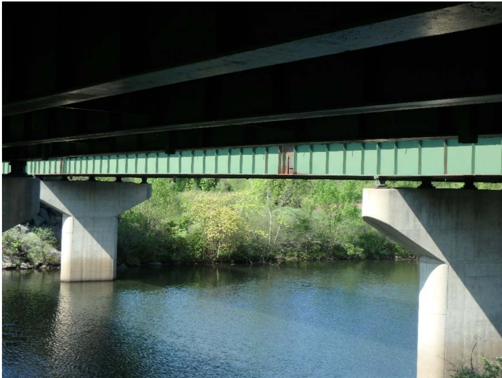
From underside of Bridge 26N Abutment #2, facing Bridge 26S
