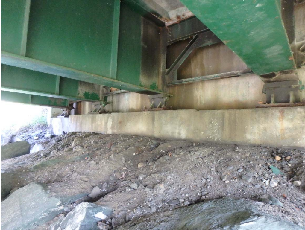
Face of Abutment #2 of Bridge 26N
