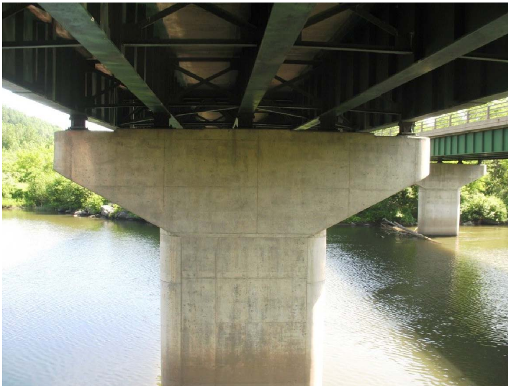
South Face of Pier #1, from Abutment #1 of Bridge 26S
