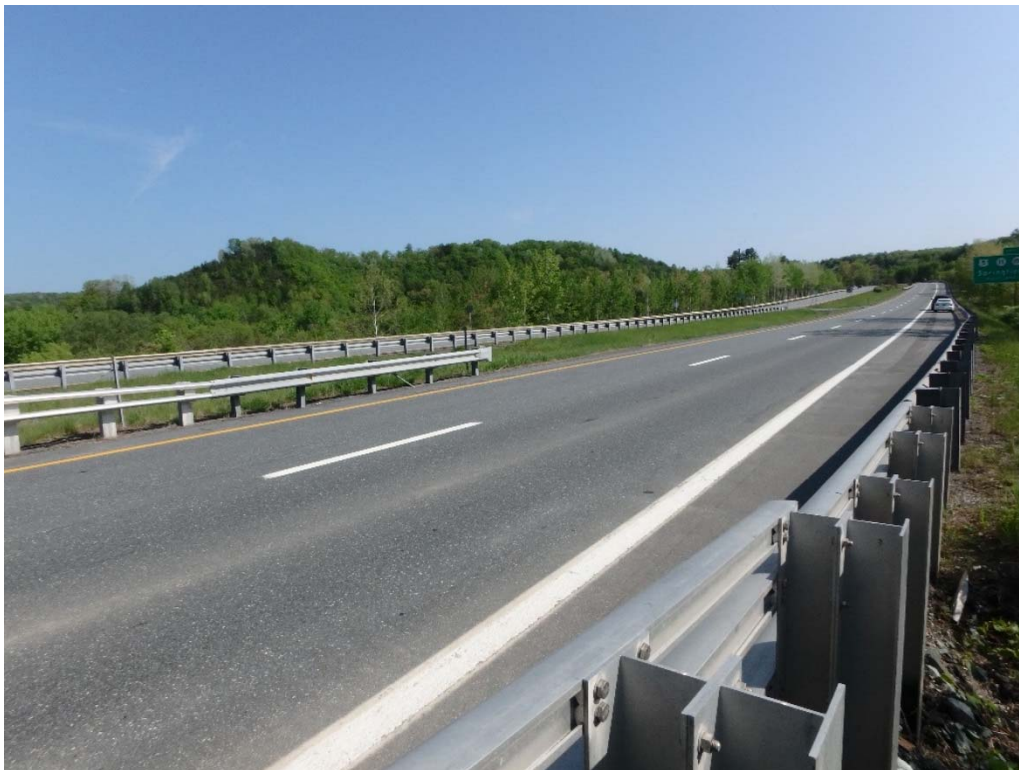
Bridge 26N, Facing South
