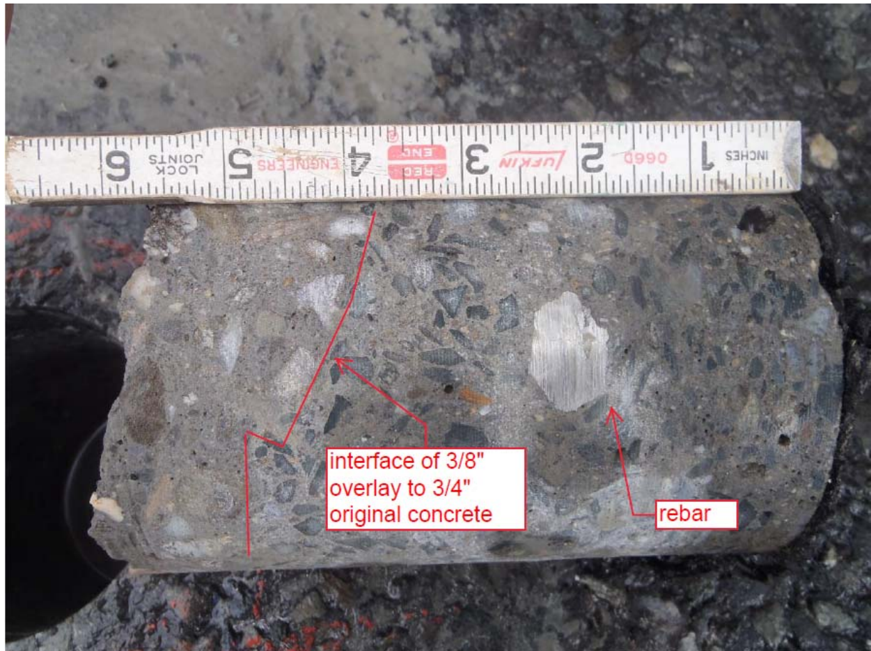
Core 2C showing interface of 3/8" aggregate concrete to 3/4" concrete.
