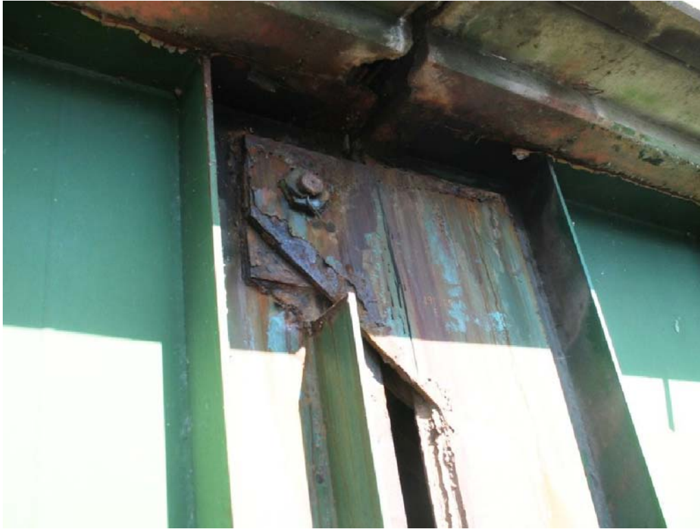
Pin Condition (Bridge 26S shown)
