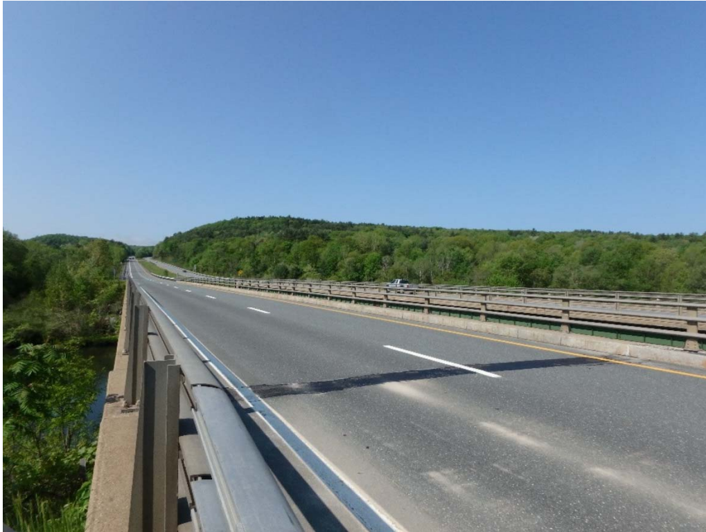
Bridge 26N, Facing North
