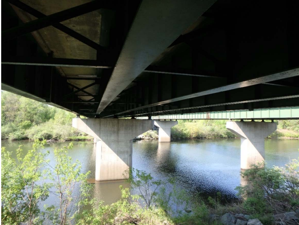
Underside of Bridge 26N, from Abutment #2
