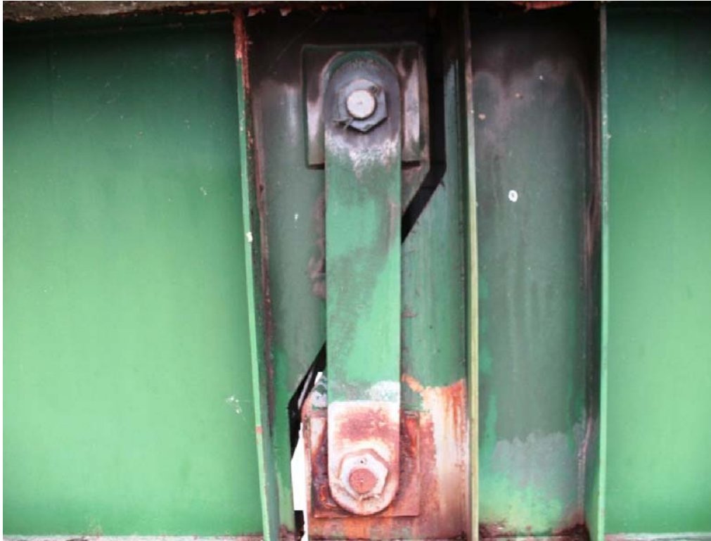
Bridge 26N Hinge
