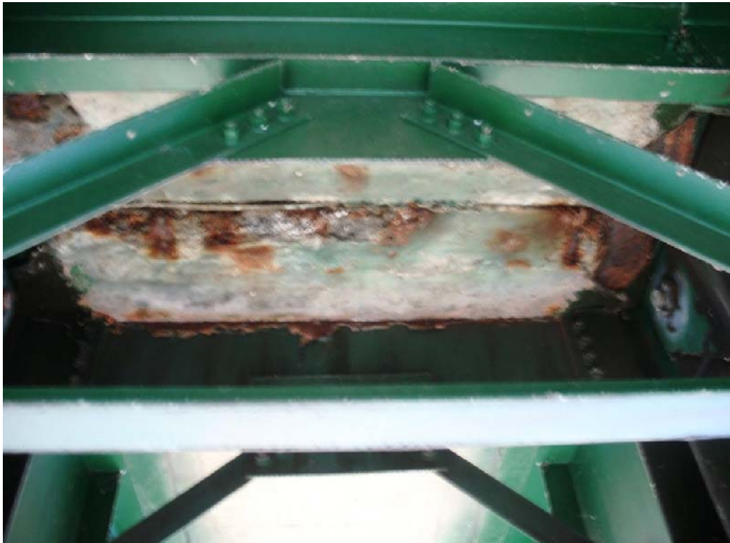
Deck Condition above Pin (Bridge 26S shown)
