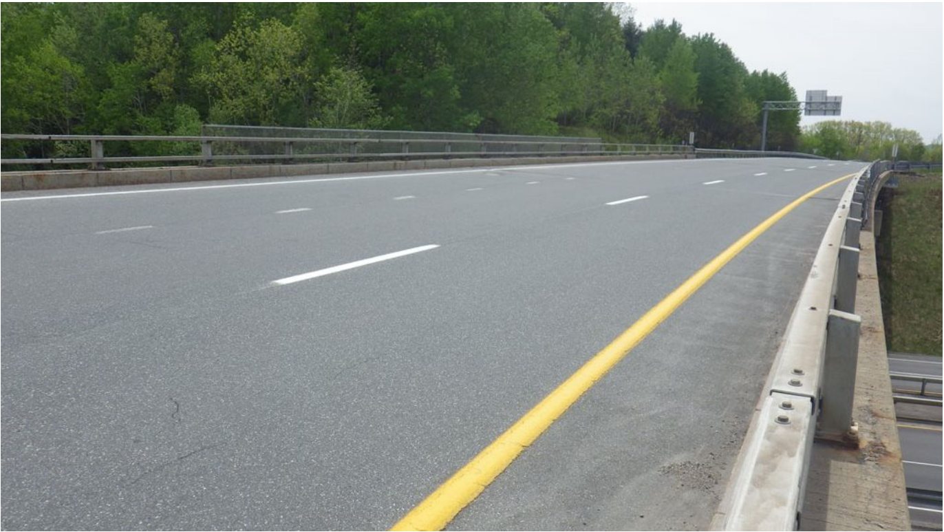
Looking South over Bridge 28N
