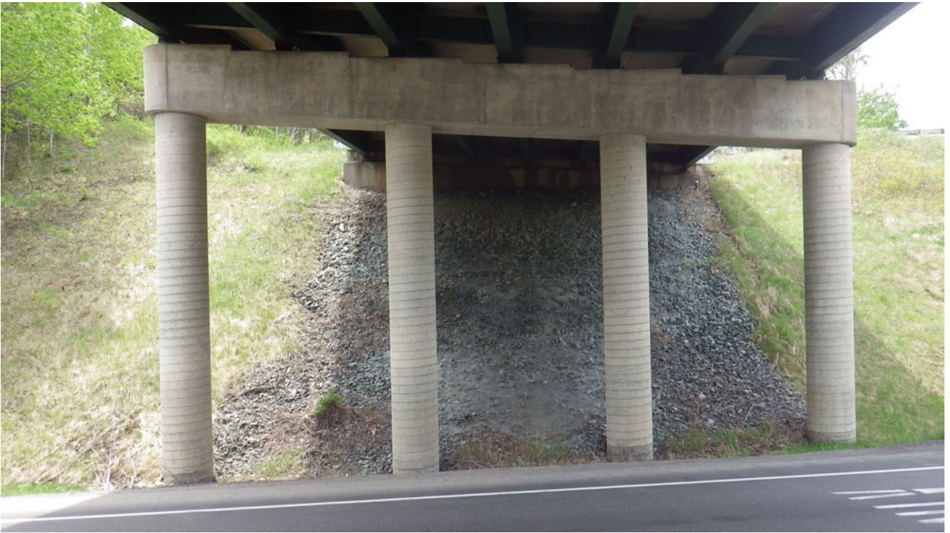
Pier column and cap condition
