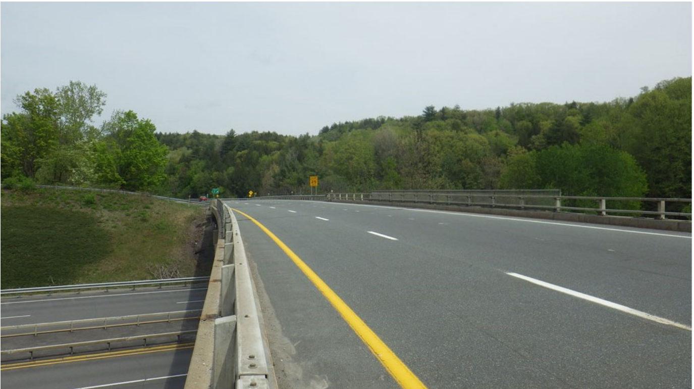
Looking north over Bridge 28N
