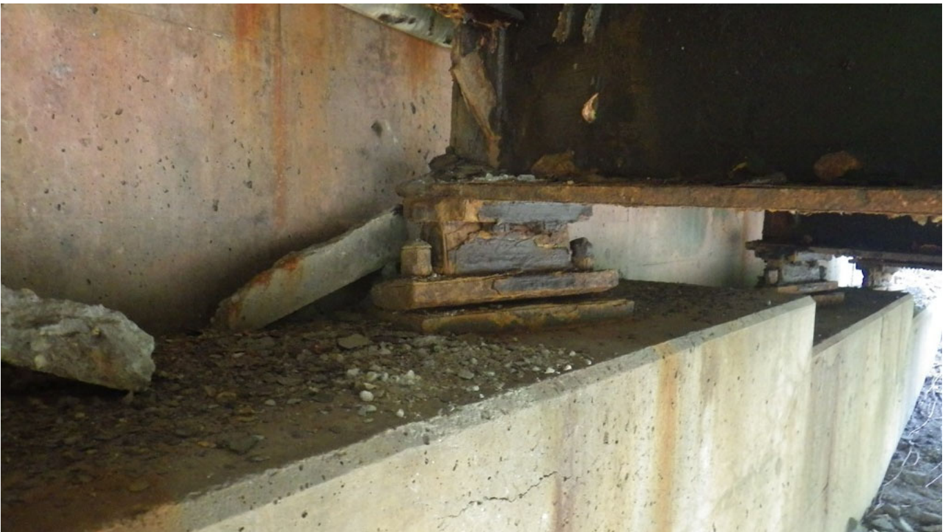
Bridge seat and bearing condition
