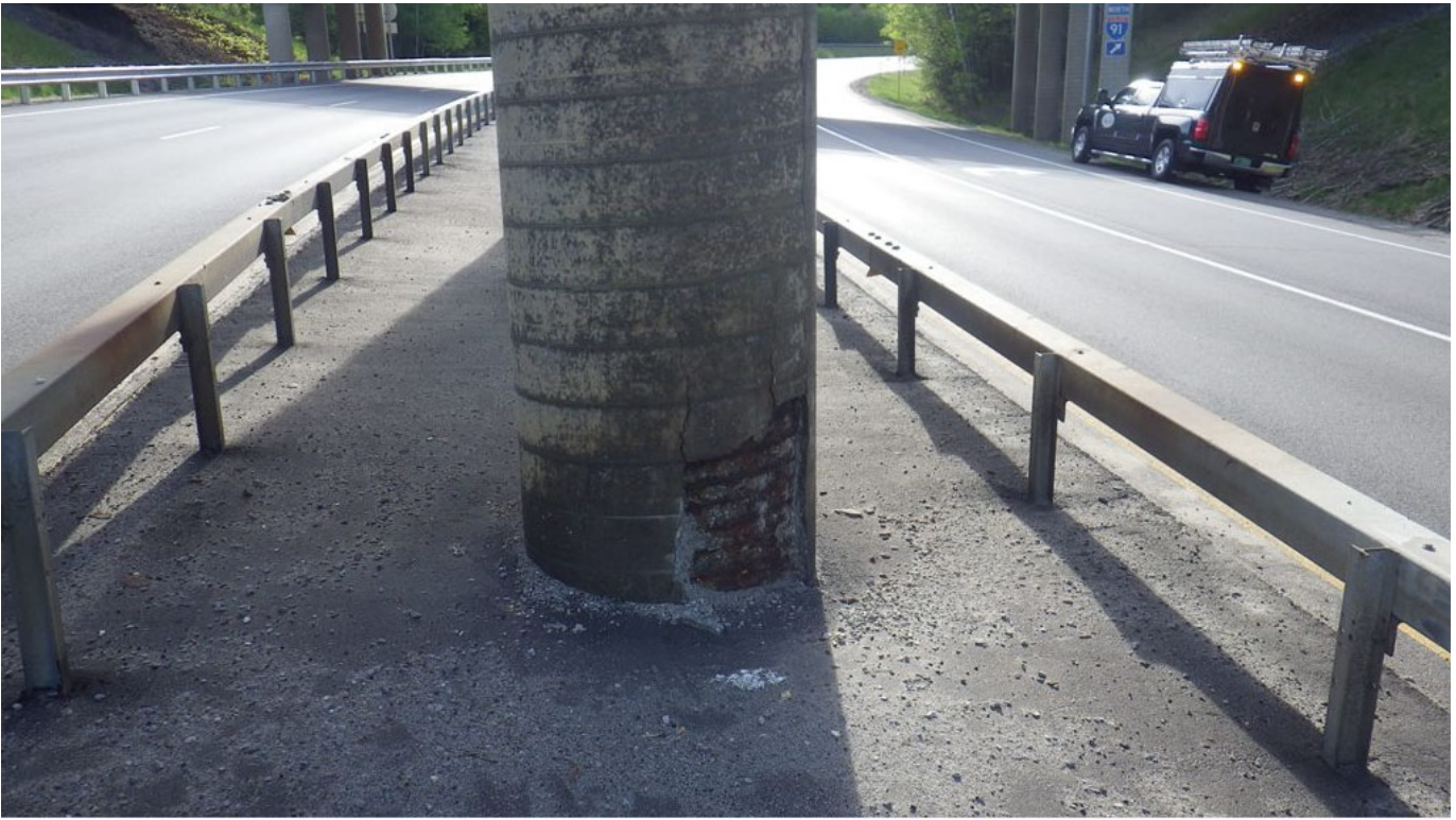
Pier column condition
