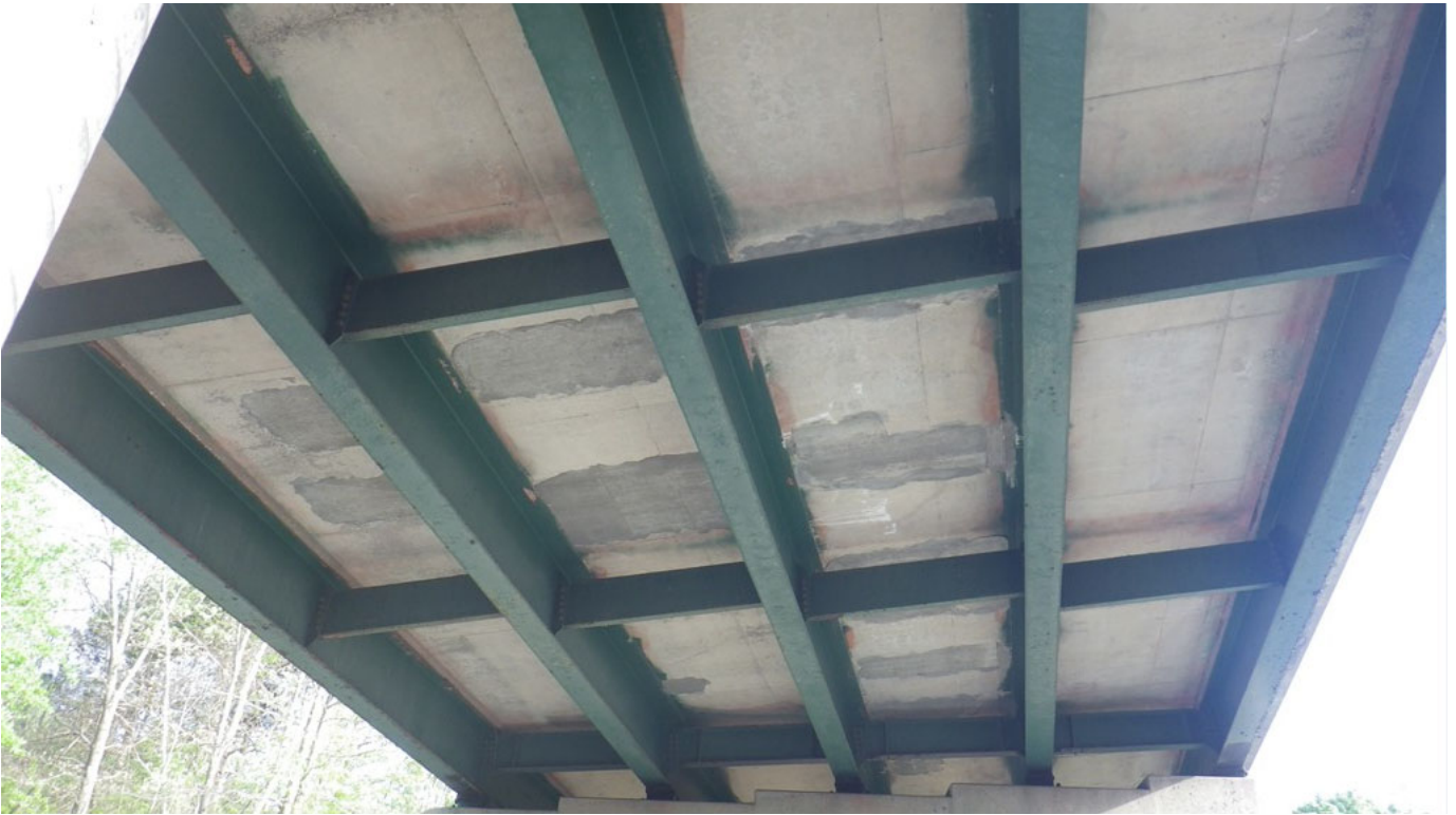
Bridge deck and superstructure condition
