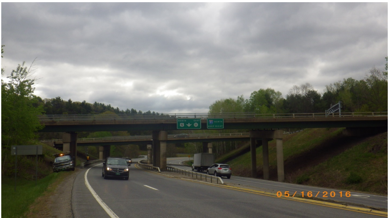
Figure 3.4: Facing east, Bridge 28 Southbound. [Inspection photo dated 2016]
