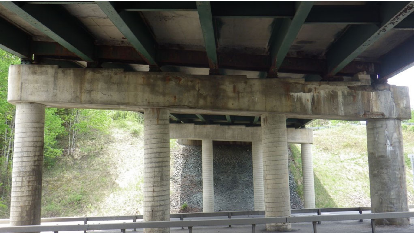
Pier column and cap condition
