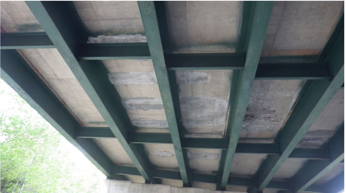
Deck and superstructure condition
