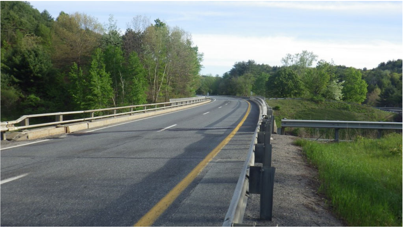
Looking north over bridge 28S
