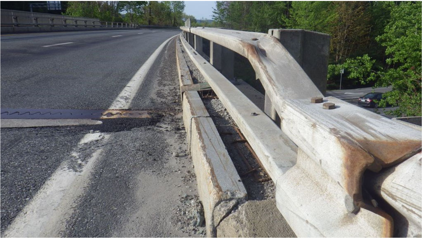
Looking South over Bridge 28S
