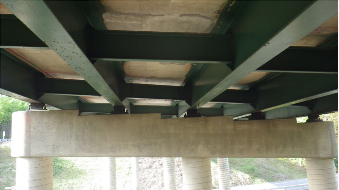
Pier cap condition
