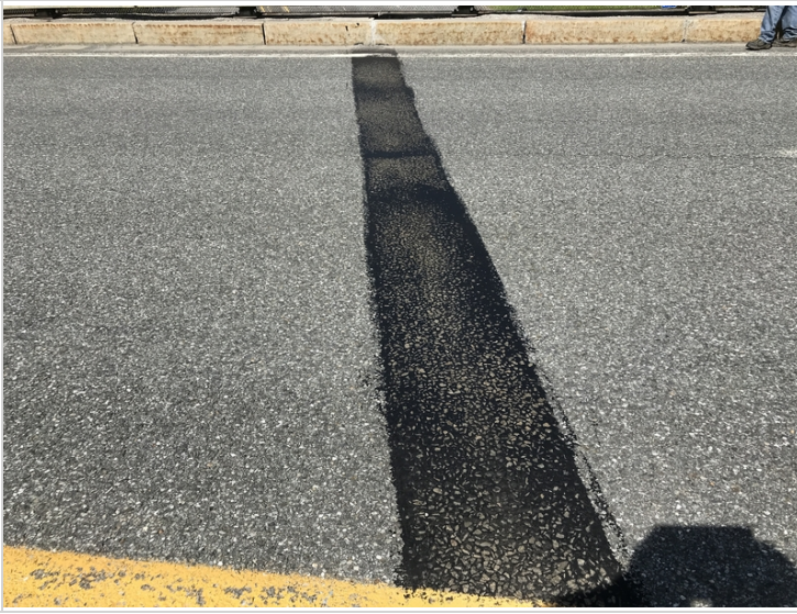
Asphaltic Plug Joint over Pier #2
