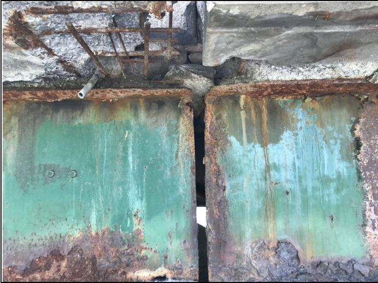
Beams #1 over Pier #2
