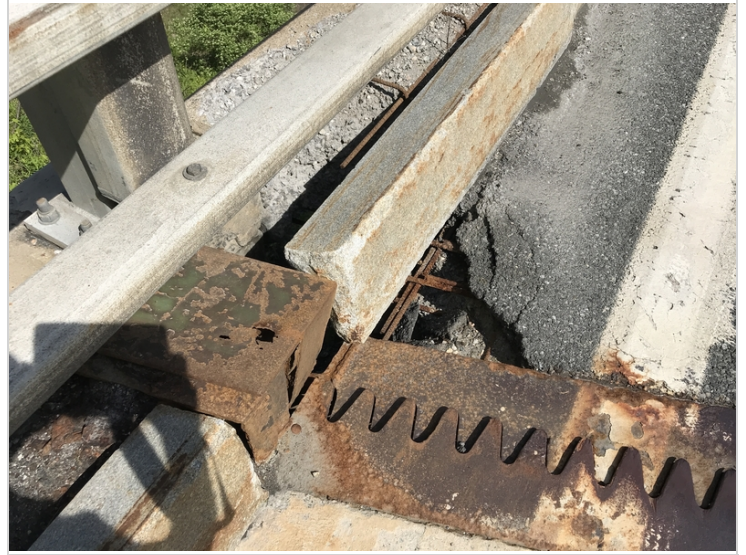
Southwest Corner of Deck at Abutment #1
