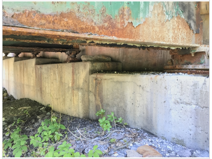
Bearings at Abutment #1
