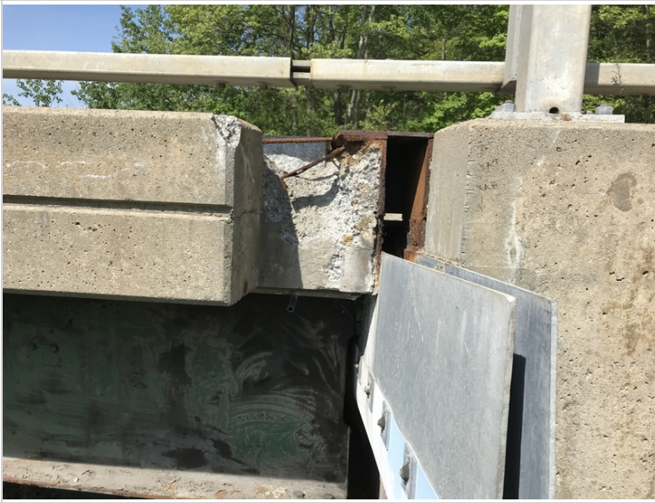
Eastern Curb at Abutment #2
