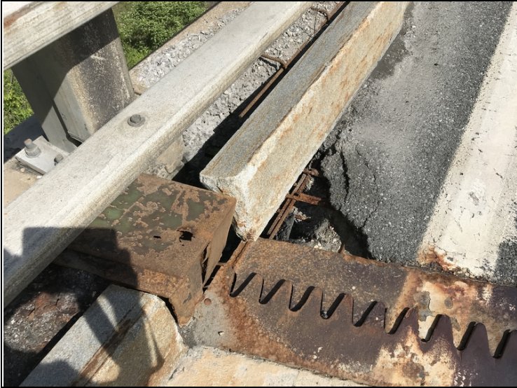
Southwest Corner of Deck at Abutment #1
