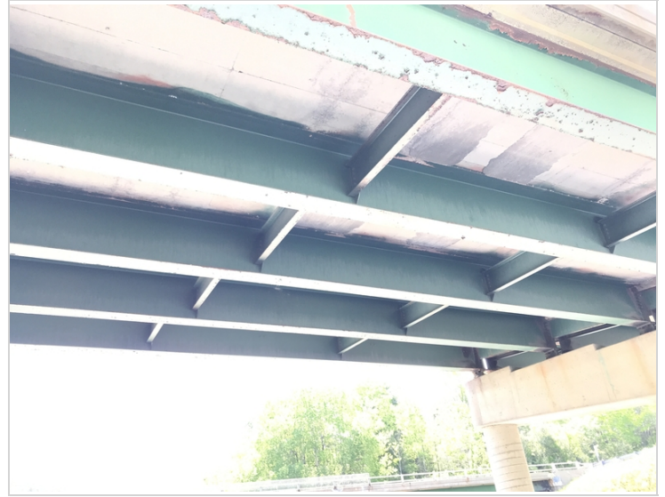
Span #3 Protective Coating
