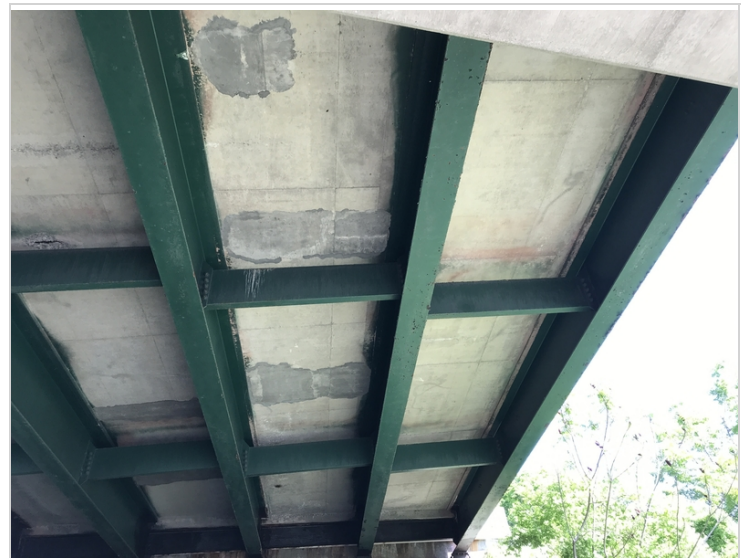
Span #4 Deck Bays 3-4
