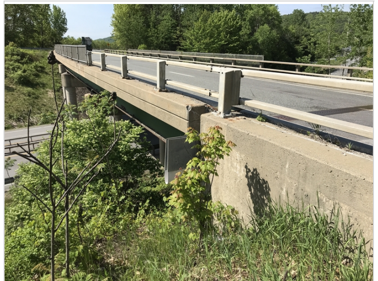
Eastern Fascia from North End
