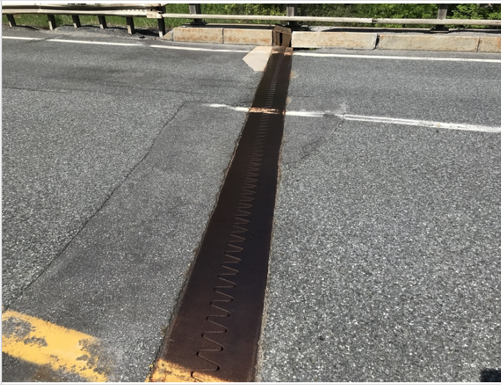
Steel Finger Plate Joint over Abutment #1
