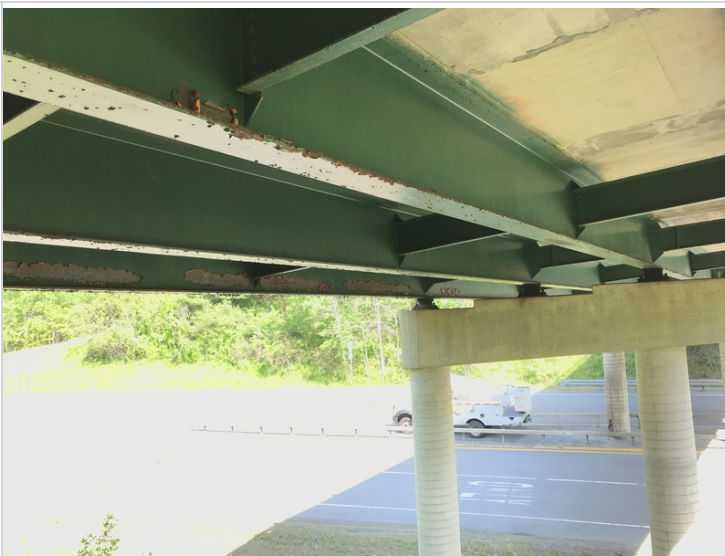
Span #1 Protective Coating
