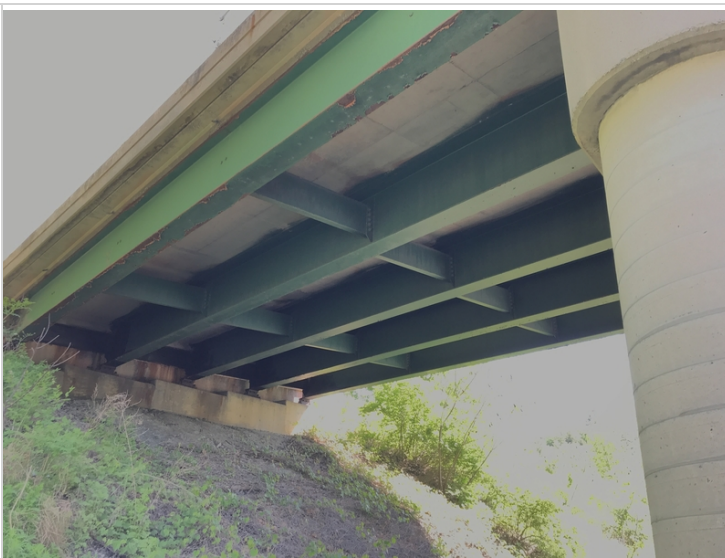
Span #4 Protective Coating
