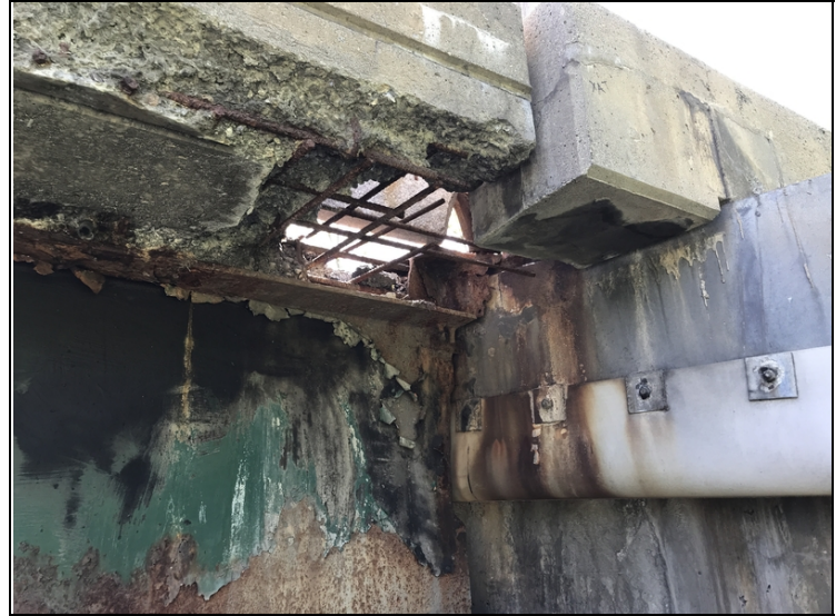
Southwest Corner of Deck at Abutment #1
