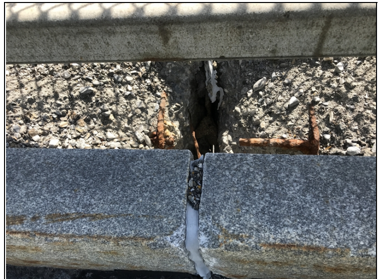
Eastern Curb at Joint over Pier #2
