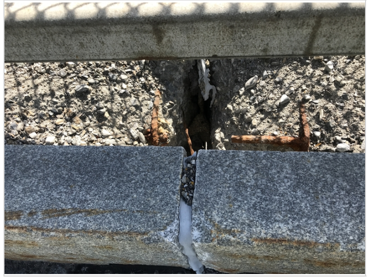
Eastern Curb at Joint over Pier #2
