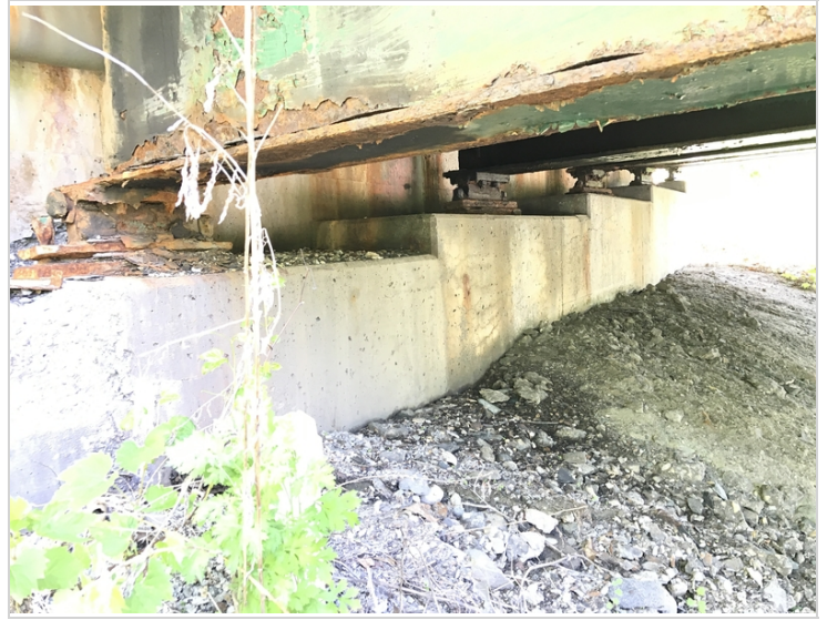
Bearings at Abutment #2
