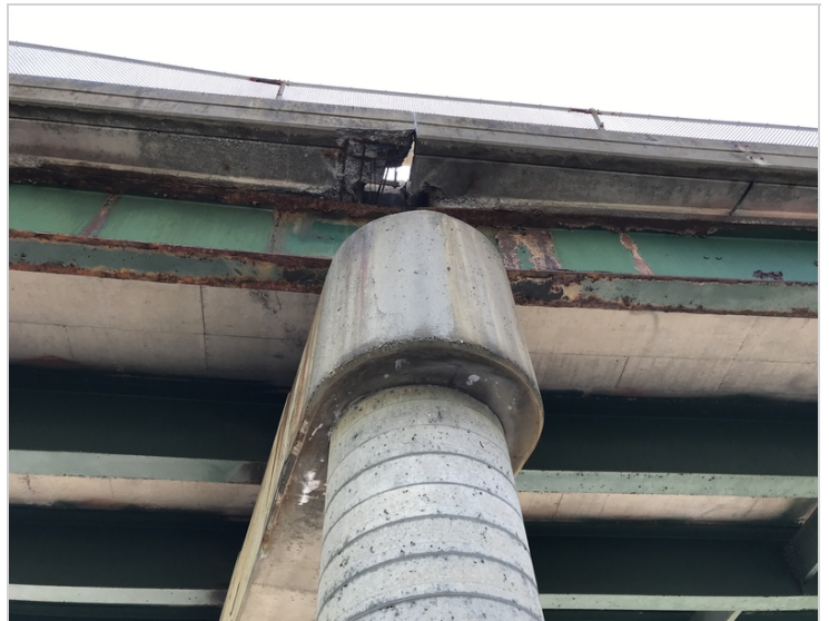
Pier #2 Joint Fascia
