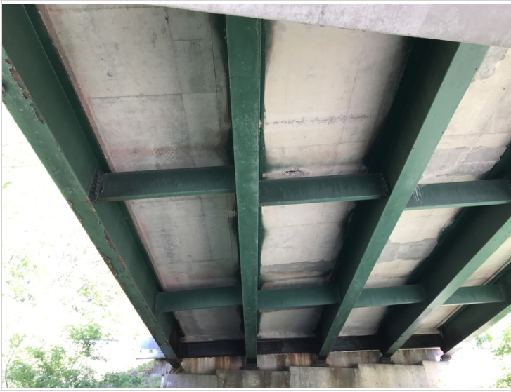
Span #4 Deck Bays 1-2
