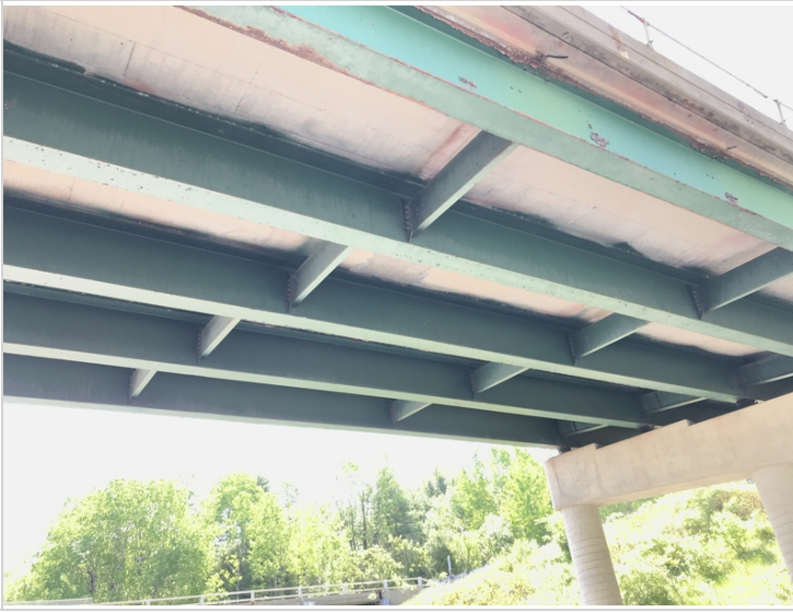
Span #2 Protective Coating
