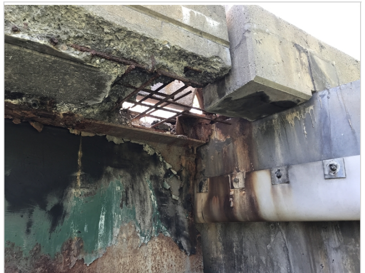
Southwest Corner of Deck at Abutment #1
