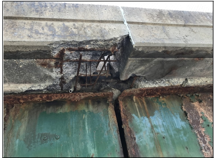
Pier #2 Joint Fascia
