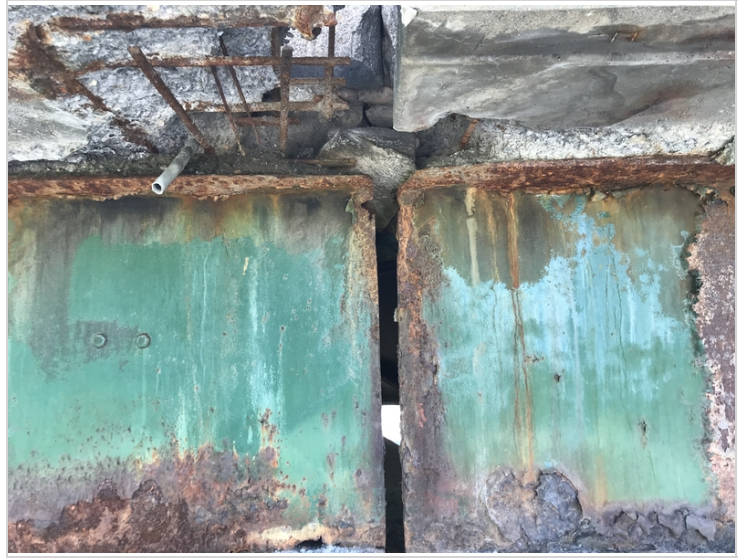
Beams #1 over Pier #2
