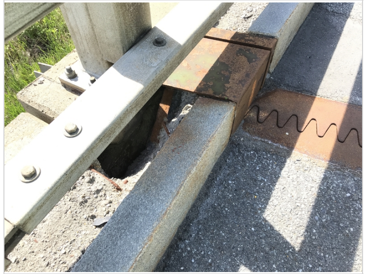
Southeast Corner of Abutment #1
