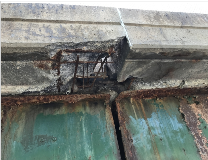
Pier #2 Joint Fascia
