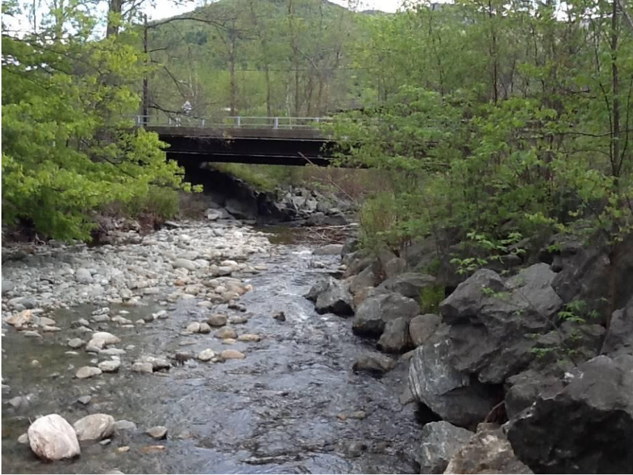
US Route 2 bridge over Joiner Brook
